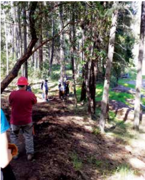
Students working on the trail after learning how to use the proper tools to angle the backslope, find the hinge point, and do the tread with a 3-5 percent outslope. The instructor, Duane Mallams (red hard hat), observes their progress.
